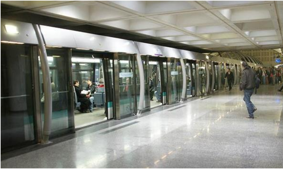
Figure E-9. Platform-edge doors
